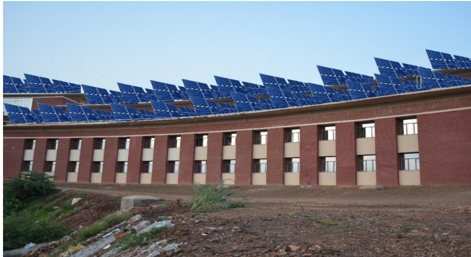
Fig 1.Set-up of solar panel
