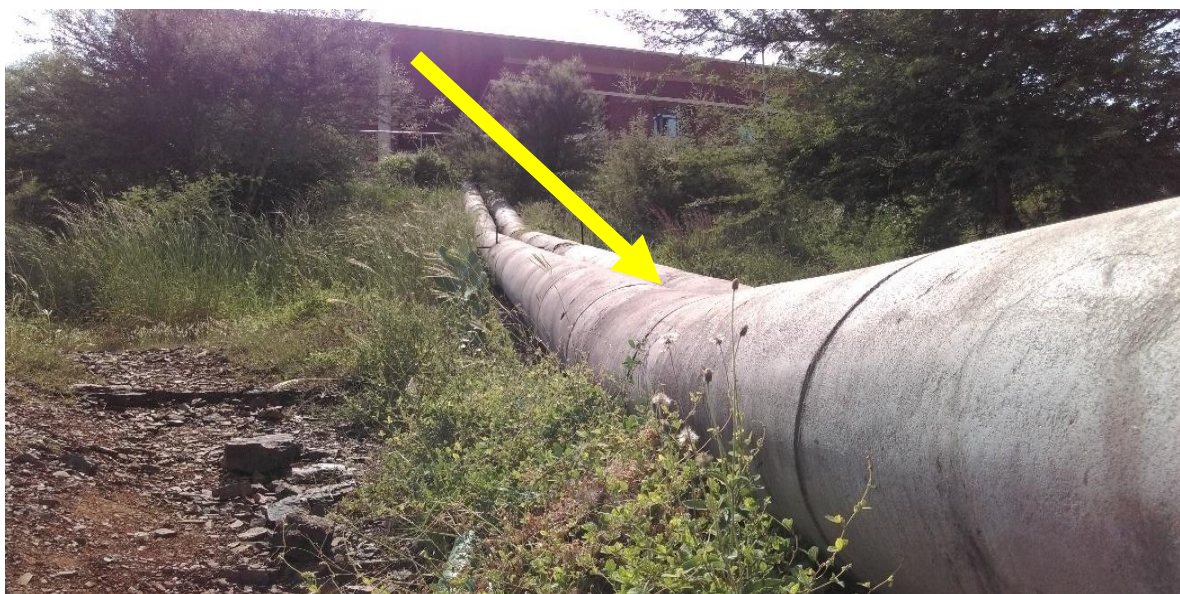
Fig.5. Set-up of pipes for running turbines
